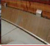
Floating Roof Seal
